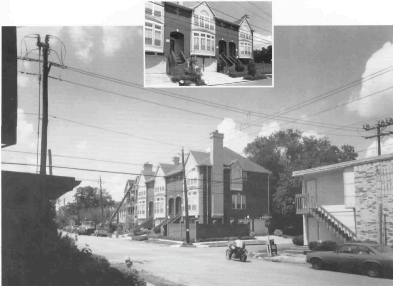
The city's interpretation of the Uniform Building Code allows townhouse developers to build three full stories without a second means of egress from the third floor, a boon to those who want to maximize square footage on narrow inner-city lots.
