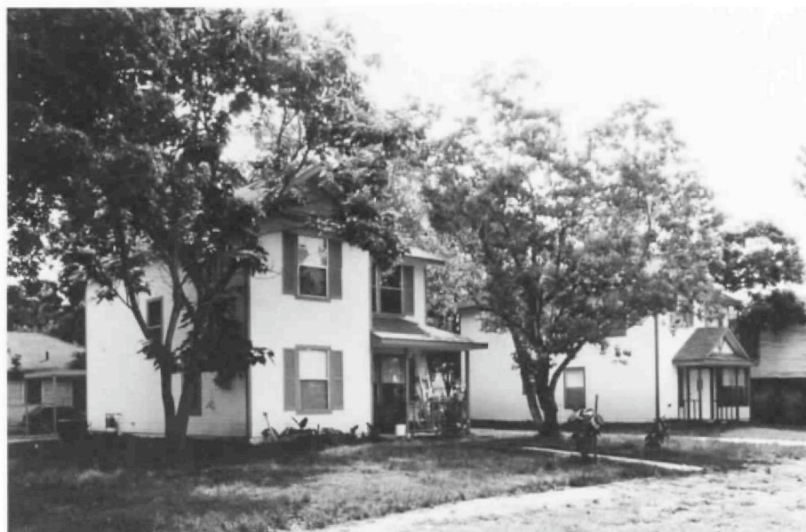
Two homes on Garrow Street (Karen Hamilton, architect), built by the Second Ward CDC: the first new housing in this neighborhood in the last 50 years.
