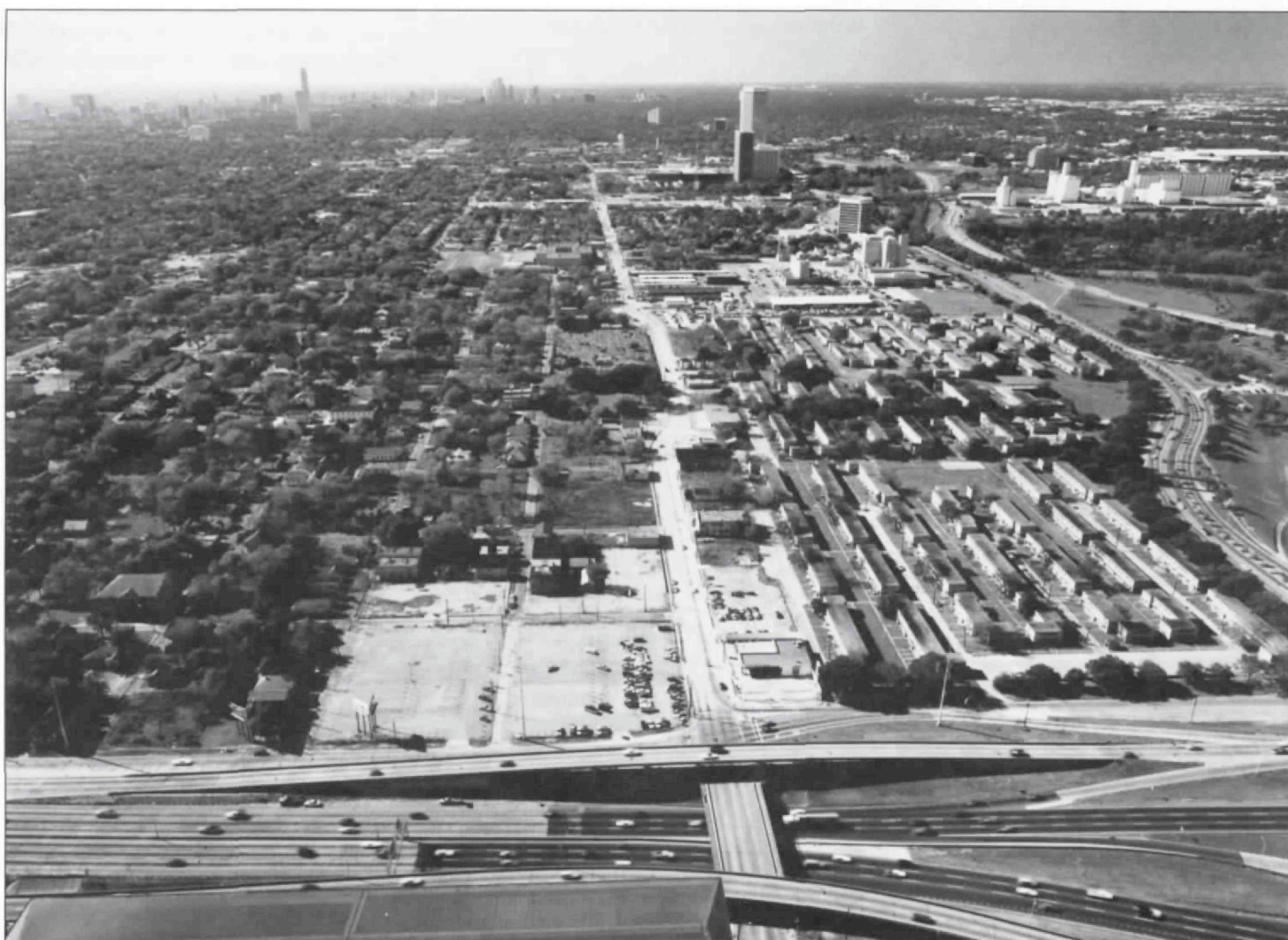
Aerial view looking west from downtown along the axis of West Dallas Avenue. Allen Parkway Village and Buffalo Bayou are to the right of West Dallas; Fourth Ward and the Freedmen's Town Historic District are to the left. The group of three towers, center top, is part of the American General Insurance Company complex, 1989.
