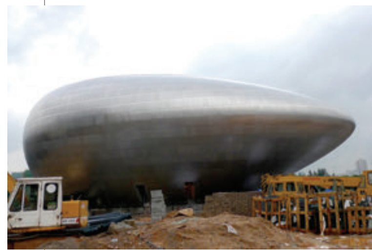
TOP Cai Guo-Qiang Courtyard House Renovation. ABOVE OCT Design Museum.
