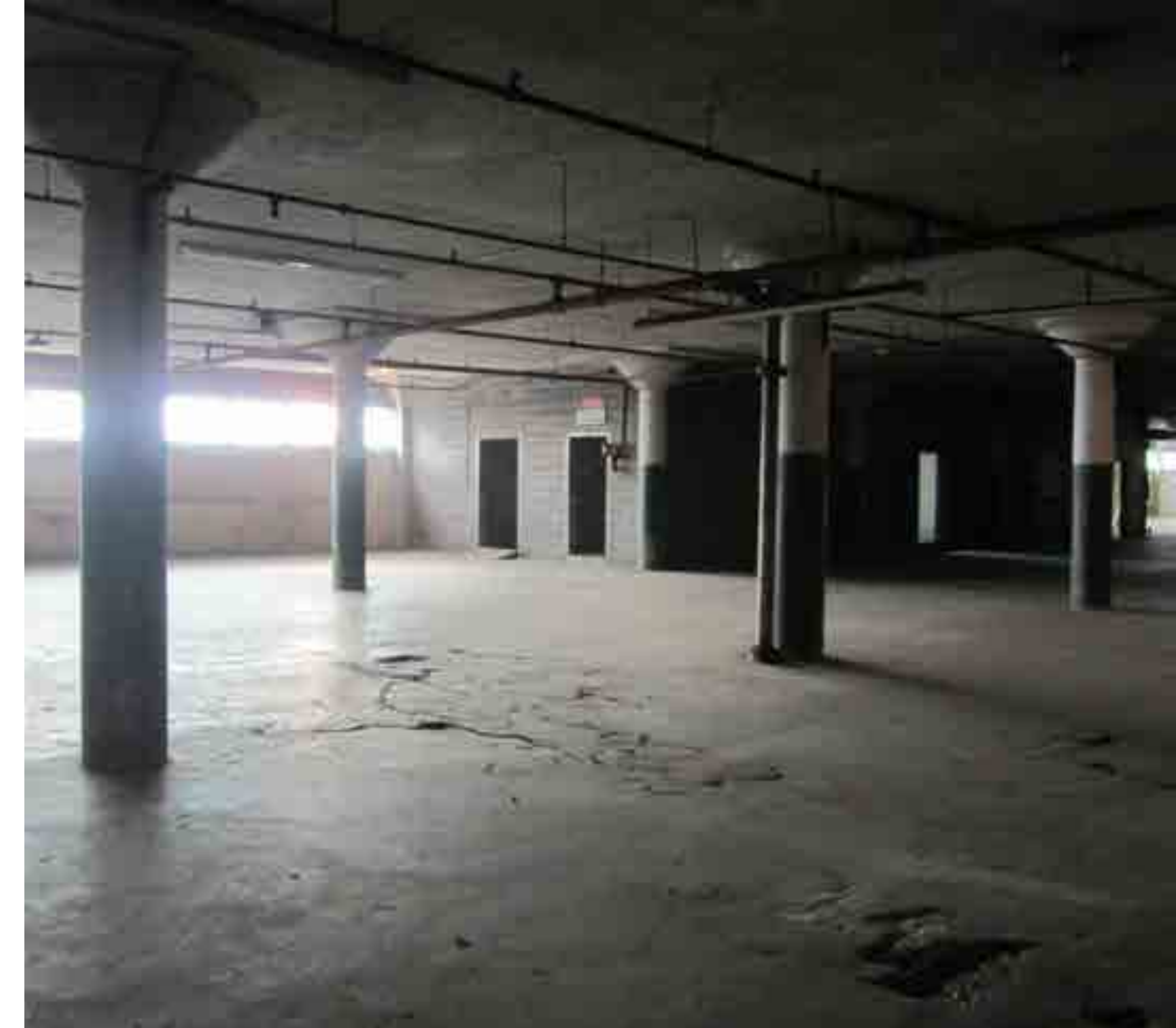
EXISTING VACANT WAREHOUSE
