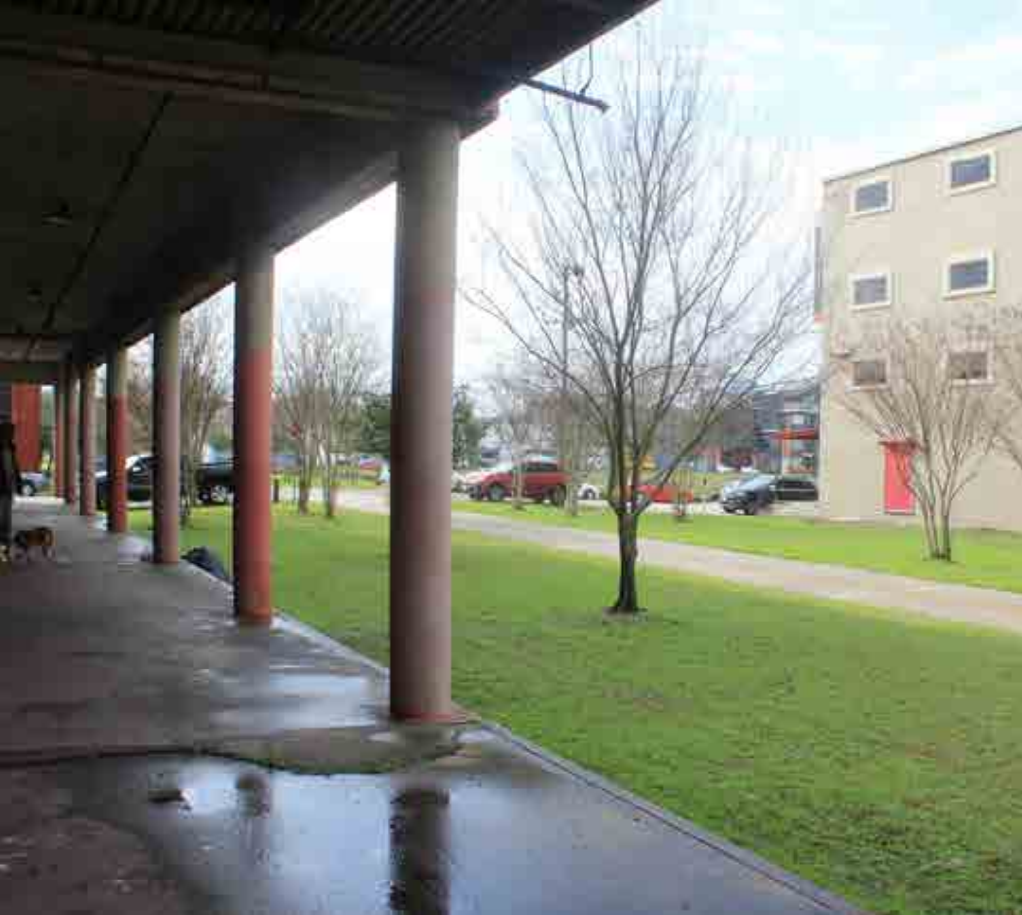
EXISTING EMPTY OVERHEAD
